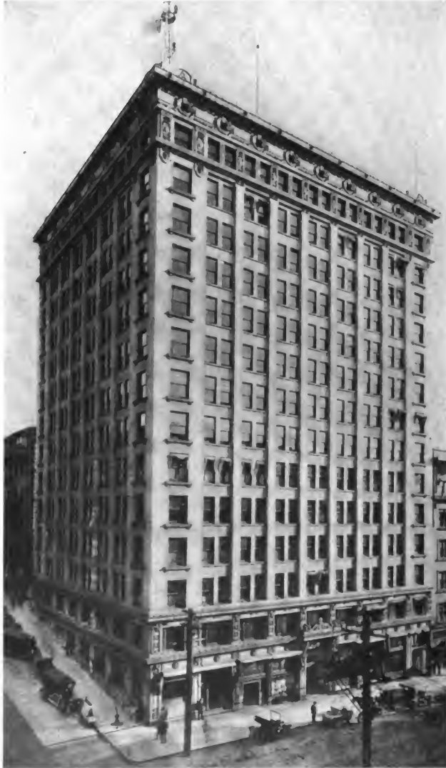
The Alaska Building—Home of the Scandinavian-American Bank.
